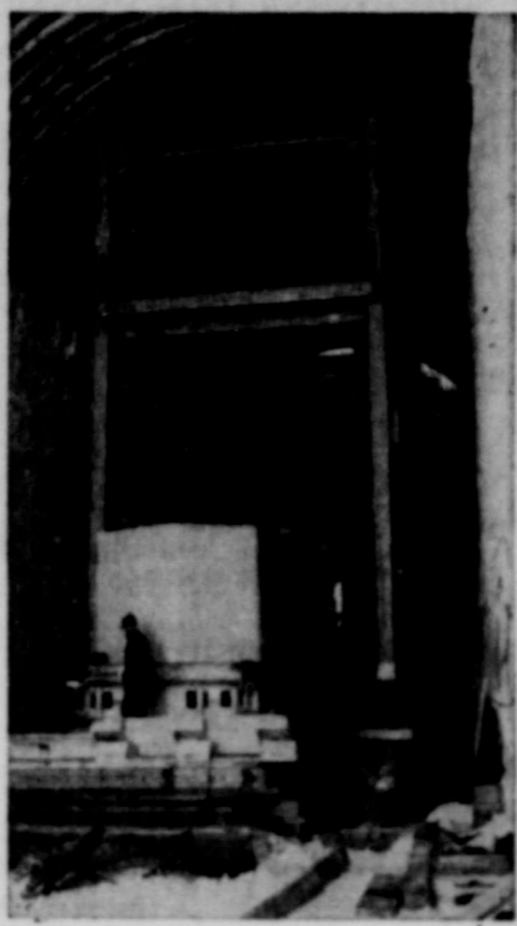
CAMP CENTURY, GREENLAND—U. S. Army Engineers install a portable nuclear power plant in a power trench built in Army's camp under the snow. Left, a component of the plant is moved down the snow drive to the entrance of the power trench. Above, a construction unit of the Engineer Corps installs part of the nuclear reactor inside the trench. The nuclear plant will send electricity into Camp Century lines for power, heating and lighting. The plant will also produce steam for melting sub-surface snow for the camp's water supply.
