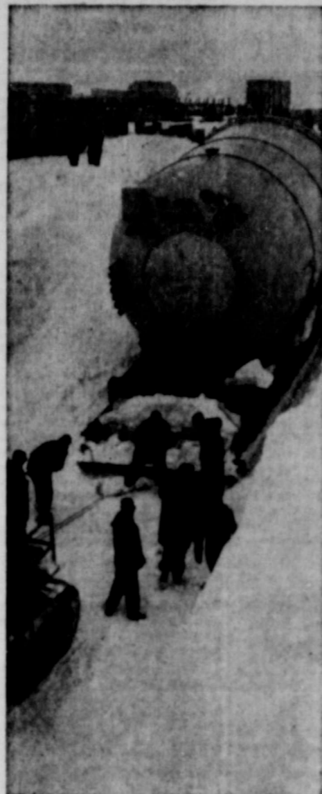
CAMP CENTURY, GREENLAND—U. S. Army Engineers install a portable nuclear power plant in a power trench built in Army's camp under the snow. Left, a component of the plant is moved down the snow drive to the entrance of the power trench. Above, a construction unit of the Engineer Corps installs part of the nuclear reactor inside the trench. The nuclear plant will send electricity into Camp Century lines for power, heating and lighting. The plant will also produce steam for melting sub-surface snow for the camp's water supply.
