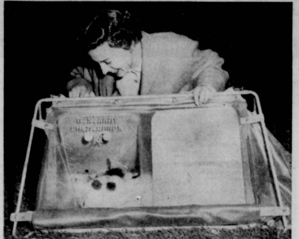
BABY'S SAFE —More than a moppel's pup-tent, the modern Army's newly-developed "infant protector" will do just that in the event of a chemical, biological or radiological attack—filtering out poison gas, bacteria and radioactive particles. A development of the Army Chemical Corps, the device offers protection to America's future generations in event of enemy aggression. Here it's being tried out by Mrs. H. A. Berrier, wife of M/Sgt. Berrier, stationed at Fort Myer, Va., and her daughter, Yvette.
