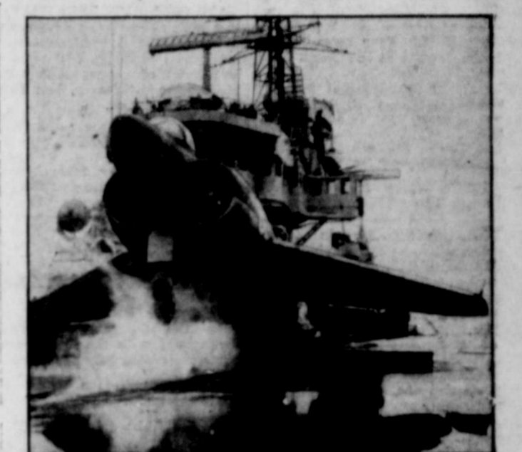
COOKIN' WITH STEAM—Vapor seeps from launching slot of a steam-propelled catapult as a Vickers Supermarine N-113 twin jet warms up aboard Britain's atom-age carrier, HMS Ark Royal.
