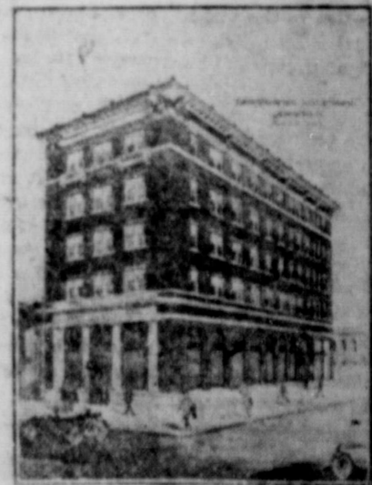
The above photograph shows the new Guaranty Bank Building now under construction on the corner of Main and Austin Streets. Plans, specifications and supervision for this building furnished by us.
