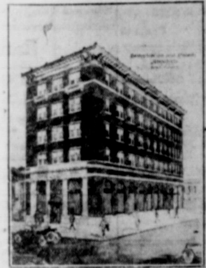
The above photograph shows the new Guaranty Bank Building now under construction on the corner of Main and Austin Streets. Plans, specifications and supervision for this building furnished by us.
