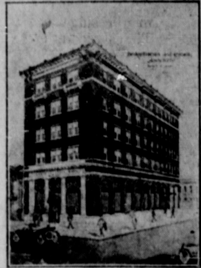
The above photograph shows the new Guaranty Bank Building now under construction on the corner of Main and Austin Streets. Plans, specifications and supervision for this building furnished by us.
