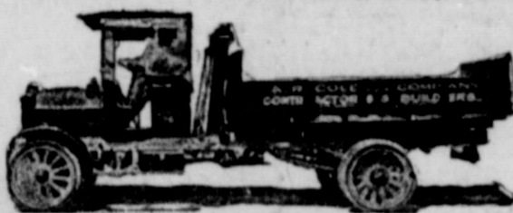
Contractors use FEDERALs to speed up the job.
