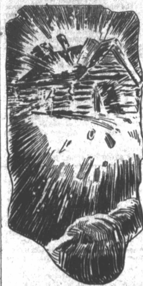
In the Flash of the Explosion We Had a Glimpse of Doors and Windows Caving In.
