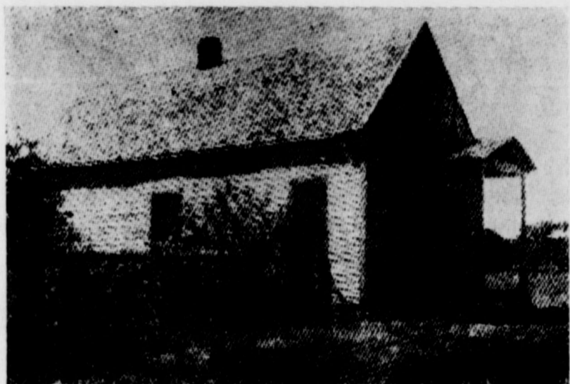
THE NEW POSTOFFICE —The building in which the postoffice at Fort Chadbourne had been housed for many years when the office was closed on
