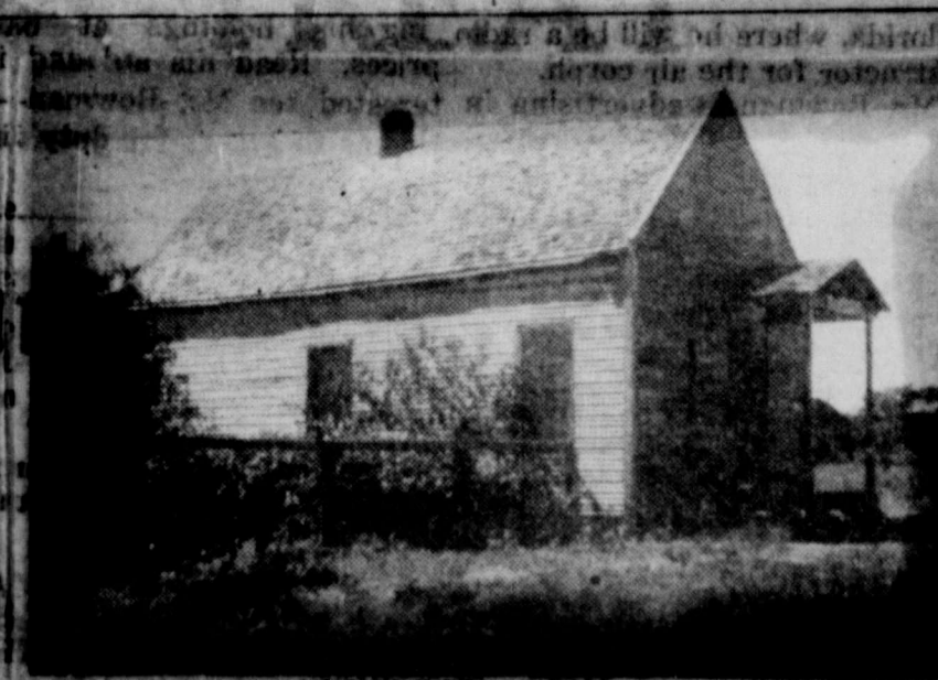
The Fort Chadbourne postoffice building in which the postoffice had been housed for many years when the postoffice was closed by the Postoffice Department on September 30, 1942, after it had been in existence for about ninety years. Mrs. Noza Hallmark was the postmaster in charge and had been postmaster since 1928. Mrs. Hallmark was the last of a succession of women postmasters in charge of the office and its affairs for more than sixty years.
