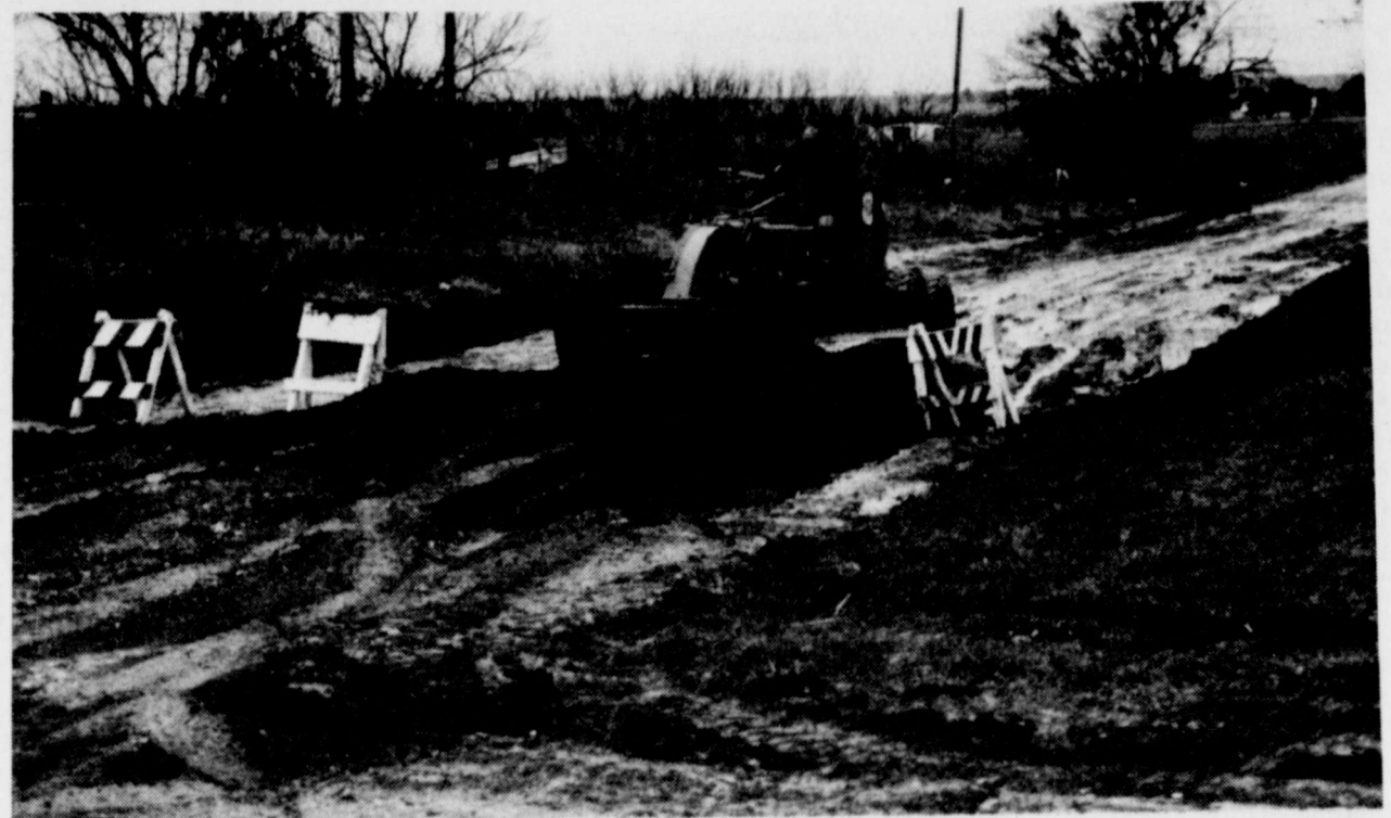
REPAIRING STREETS — Employees of the City of Winters were out in full force this past week repairing damage to city streets caused by excessive rain. In picture above, superintendent Charles Grenwelle fills in Truett street with hard base and caliche.
