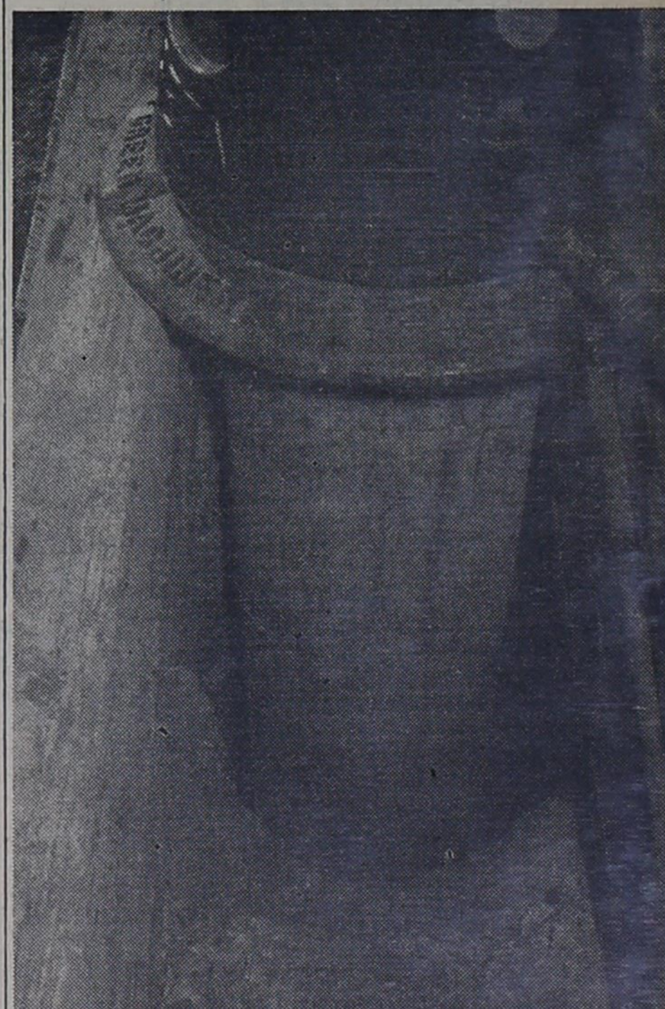
IT COULD HAPPEN IN BOVINA — This graphic illustration of carelessness shows a gaping hole at the newly-drilled water well west of the baseball diamond. There's plenty of room for a child to slip into the hole, bringing about another casualty on the order of the nationally publicized tragedy in California several years ago, when a six year old girl fell into a well shaft. However, Henry Minter and the photographer placed a temporary covering over the hole to eliminate the hazard.
