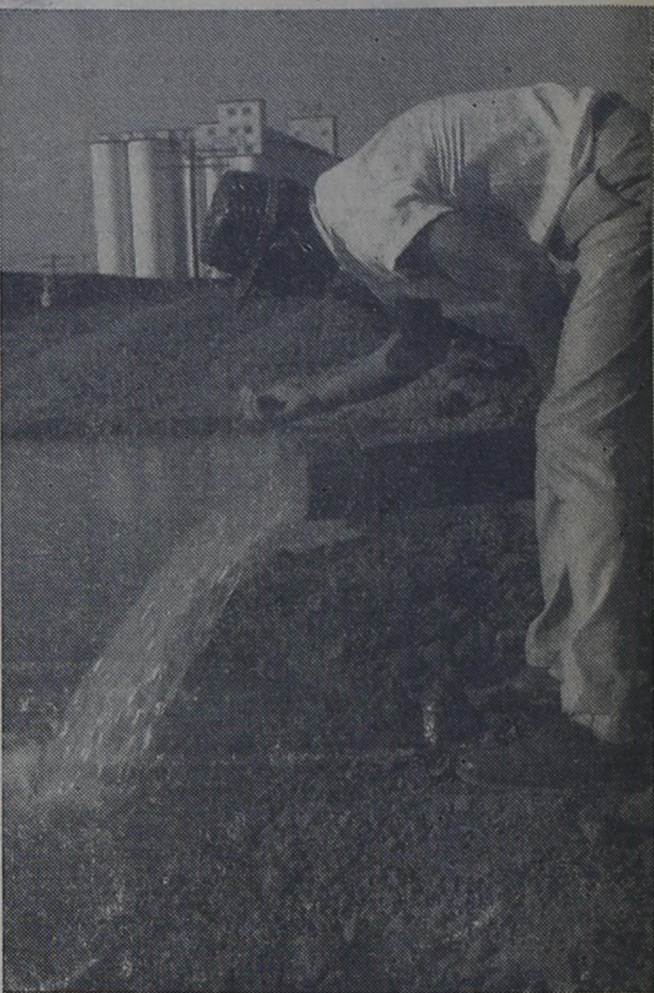
WATER AND SAND — Bovina City Clerk Henry Minter catches a handful of water mixed sand at the newly-drilled water well for the city water system. The well was still pumping sand after five days of pumping.
