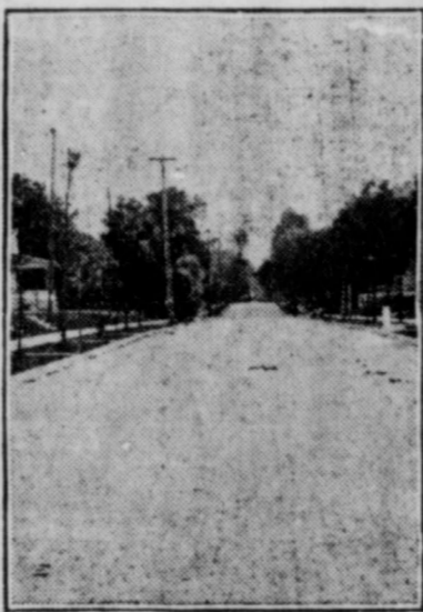
From Good Roads Magazine, New York. WELL BUILT BRICK ROADWAY.
