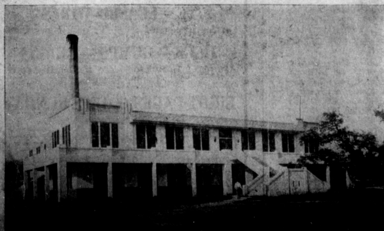
Subistence Building (Opposite Kerrville Memorial Sanatorium)
