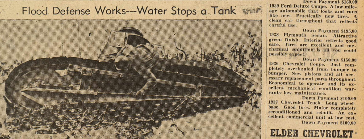
Here's what happens to a tank when the dikes are opened in Holland and the water comes pouring out over the land. Dutch tank shown above was more than half submerged in flood defense test.
