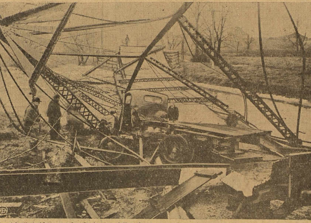
Frankfort's bridge—not London's—has fallen down and the light one and a half-ton truck, shown in the foreground of the above picture, caused it all. When the truck, driven by Landis Thompson, Sedalia, Ind., hit an end support, the entire bridge collapsed leftward.
