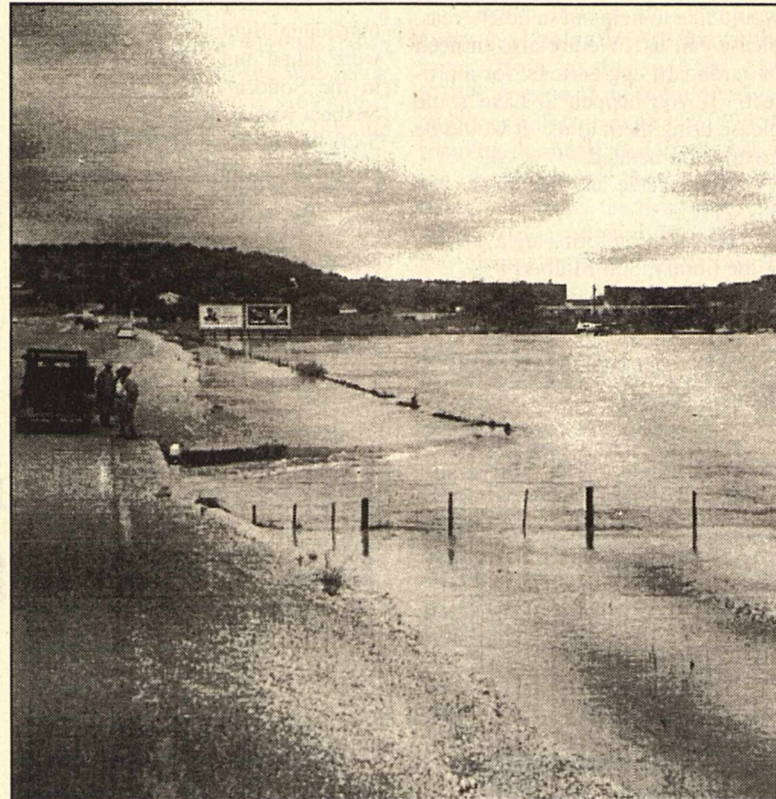
October 1957-Looking west over the south end of the Sonora Air Strip after 4-6 inches of rain fell on the 1700 acre watershed. Photo by E.B. Keng
