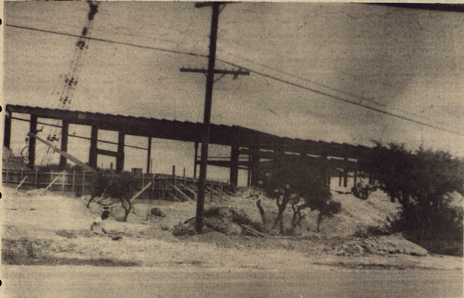
The construction for the new high school is well underway as
