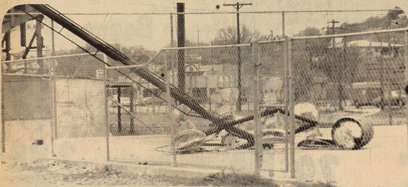
The overhead light at the Sutton County 4-H Arena is no longer overhead, as is seen here. The exceptional wind velocity last Friday in some cases did almost as much damage as did the hailstones. This metal pole was snapped almost in two about halfway down the pole. [Photo by Kay Holdridge]
