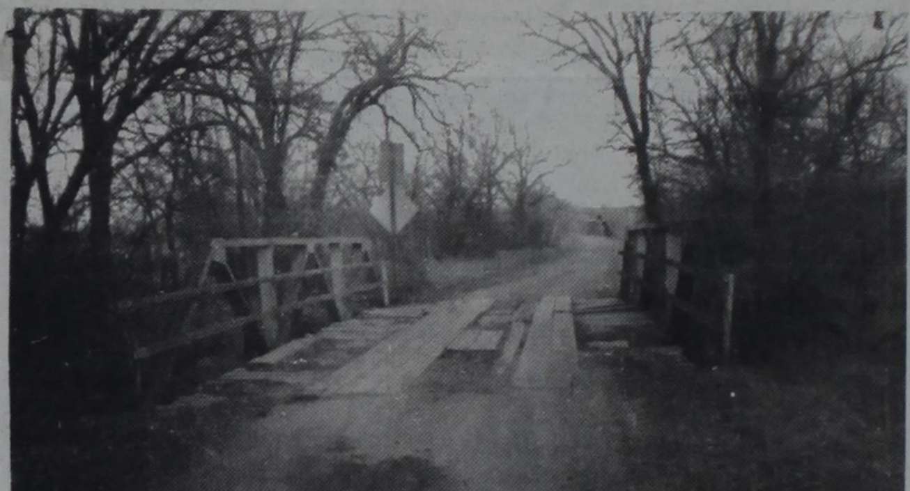
Goodbye, old bridge. This wooden bridge has seen a lot of traffic since it was built about 80 years ago. This picture was made in January of this year, the day before it was torn down for a new concrete structure on CR 180, Pct. 4.
