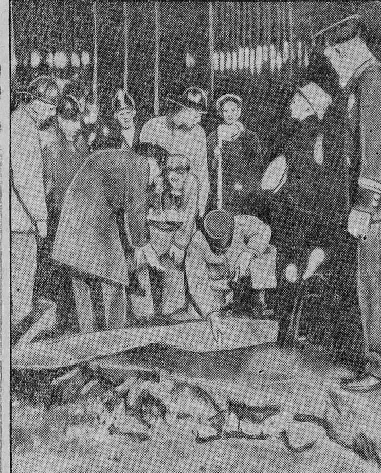
Police and firemen are shown here examining the debris after an underground explosion in front of a Los Angeles theater injured 31 persons and rocked the theater as well as other nearby buildings. The explosion was believed to have been caused by ignition of sewer gas. The performance was attended by a number of film stars and the explosion took place shortly before they were scheduled to leave the theater.
