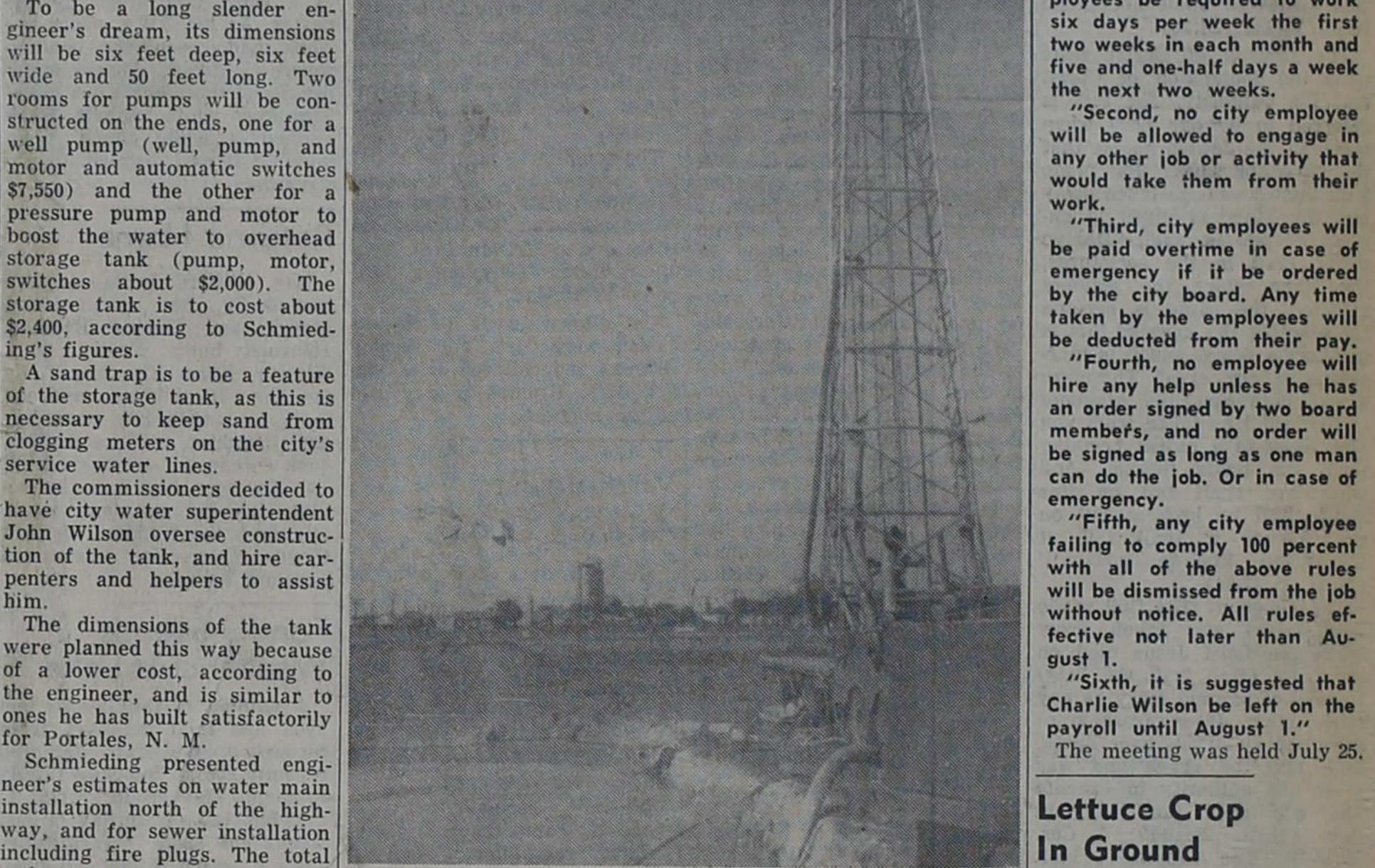
NEW WELL for the city of Bovina is almost completed. The depth was about 225 feet Tuesday morning. A water storage tank will be constructed at the location after the well is finished.
