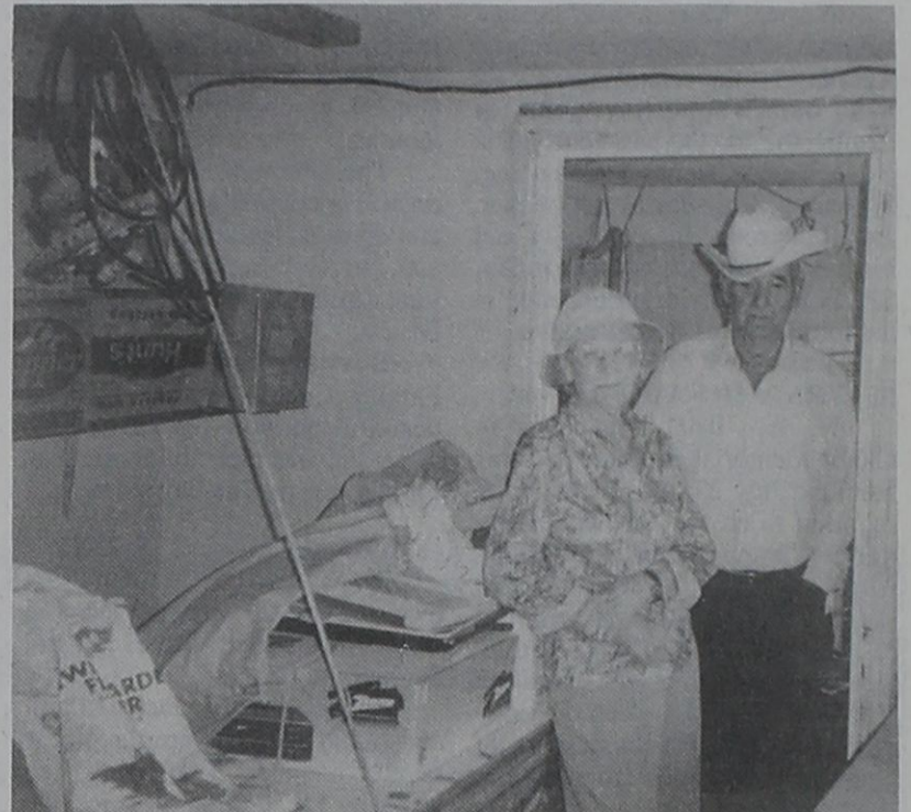
WHY? THEY ASKED..... Erma and Carl Schrader survey water damage in their storage house. Vandals left a sprinkler running inside the building and flooded it.
