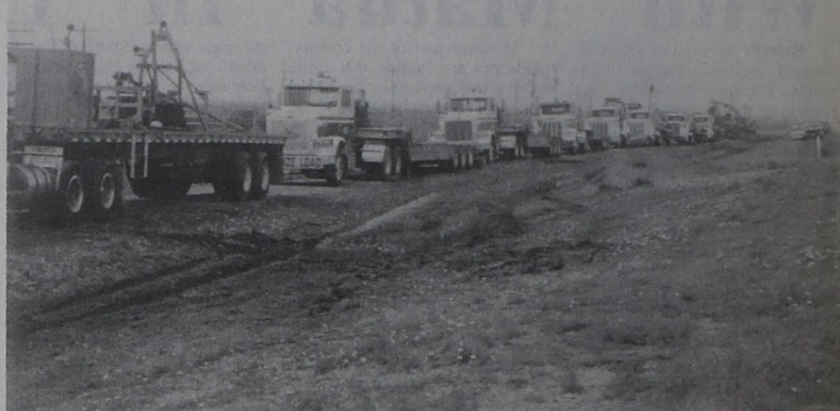
WIDE LOADS..... This convoy of wide horsepower was used to bring the huge track moving cranes in last week as work continues on the Santa Fe Railroad construction.
