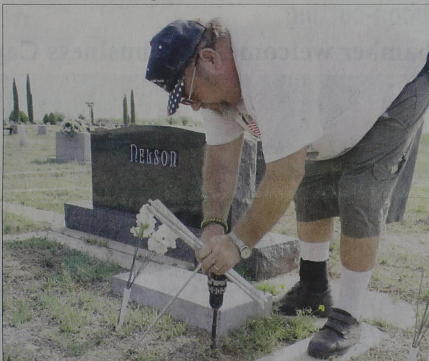
Anna Gibson/The Post Dispatch VFW Post 6797 member J.W. Jolly drills a hole for a U.S. veteran grave marker at Terrace Cemetery in Post. The markers were installed last weekend as a way to mark the graves of local veterans.
