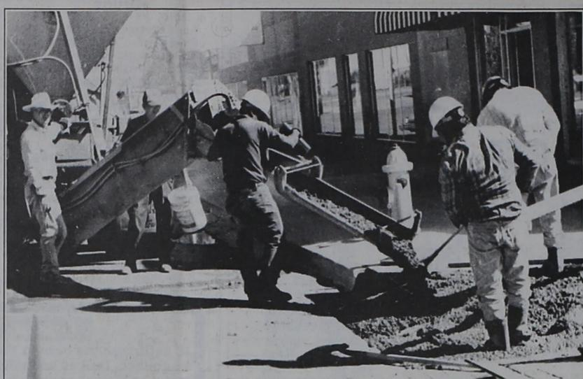
Jimmy Redman pours the concrete on one of the more than 40 ADA Wheelchair ramps being constructed with in Post's City limits. Redman has the contract for all the concrete. The labor is being furnished by Texas Department of Public Safety and Transportation.
