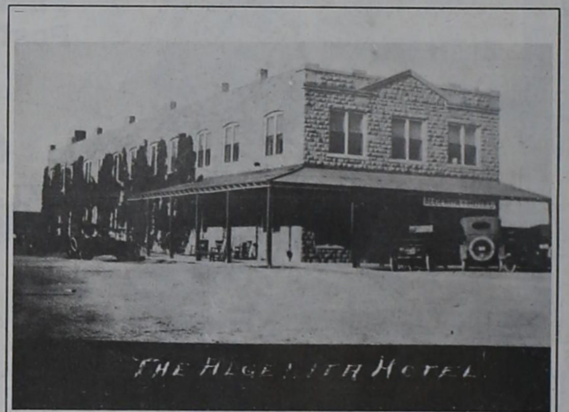
The Algerita Hotel was finished in 1908. The building was erected from native stone quarred from Alexander's Quarry. The stone quarry was discovered when a road was blasted down the caprock in order to move the city to its central location. The hotel boasted 30 rooms, a barber shop, fine food and water closets with running water. C. W. Post oversaw every step of the hotels construction, including setting up the menu.
