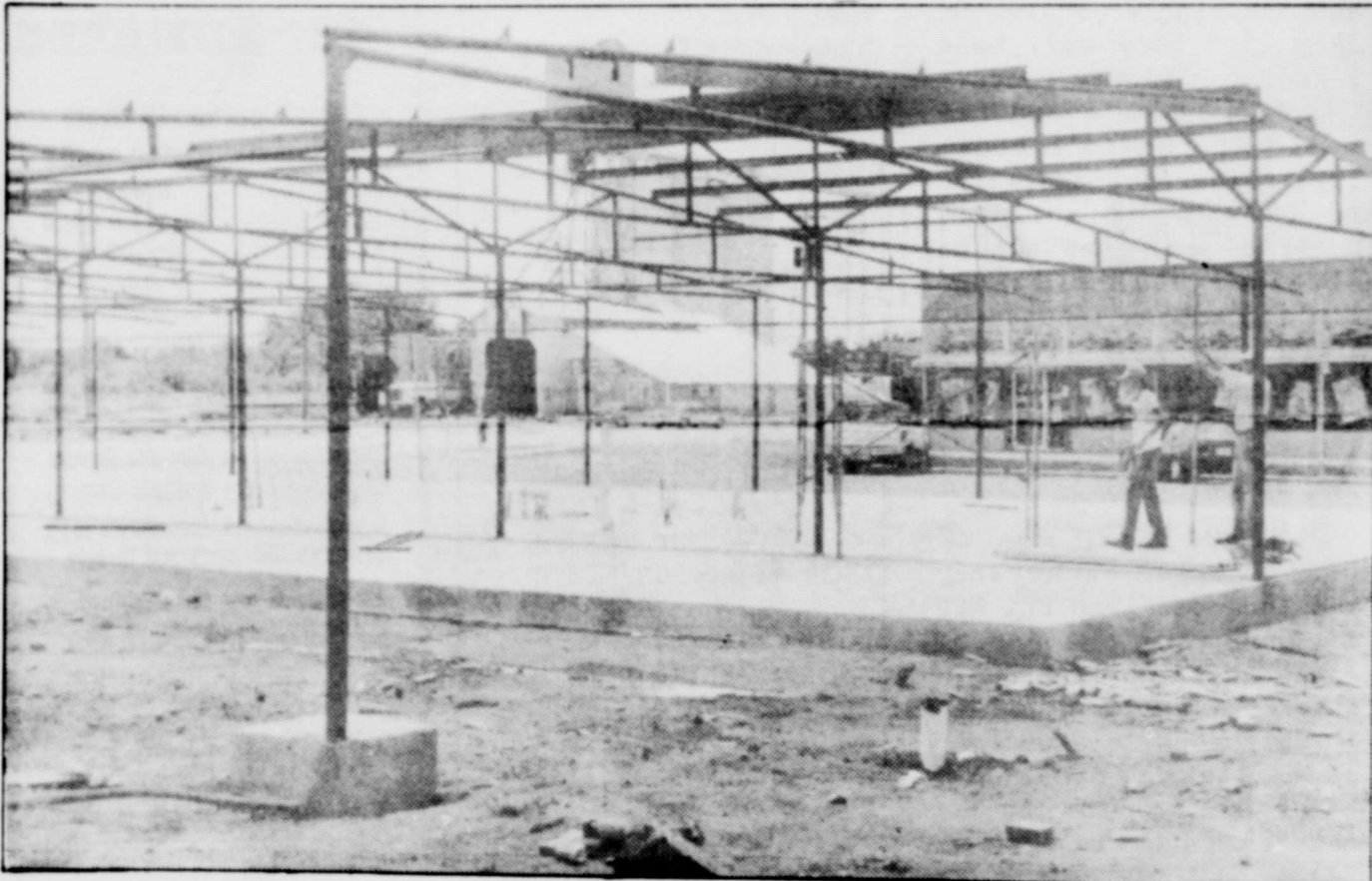
Work is moving right along on Merkel's new City Hall. Adding metal "sk-
