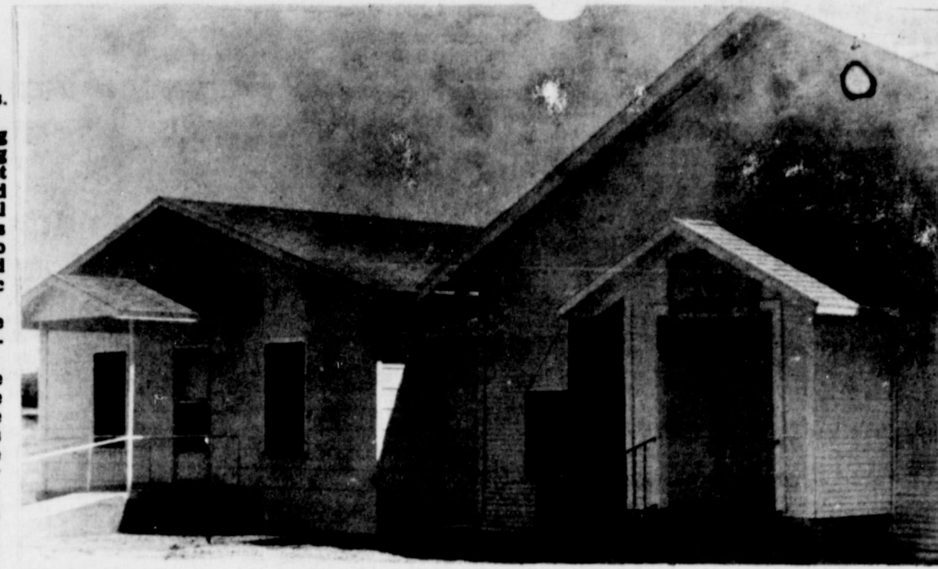
The Tye Senior Citizen's Building has been completed. The building was constructed by volunteer labor from the Tye Community. (Staff photo by Cloy A. Richards)
