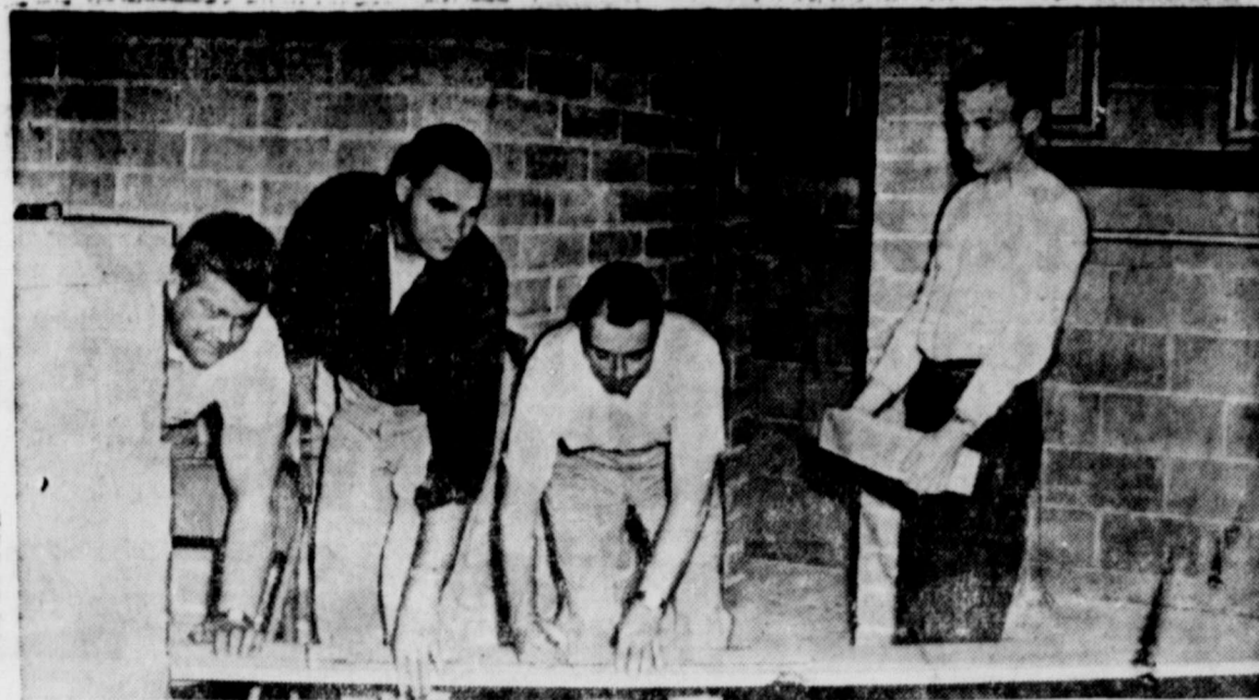
JAYCEE SHELTER project, part of the organization's nationwide "Operation Survival," takes concrete form as Blue Earth, Minn. Jaycees construct a 4-person fallout shelter in the city hall basement. This is one of a variety of permanent or temporary display shelters built by Jaycees in cooperation with civil defense in communities across the nation. Each of the 3,900 Jaycee chapters in the United States is being encouraged to participate in the program to stir public interest in fallout shelter construction in every community across the Nation. (Fairmont, Minn., Sentinel Photo)
