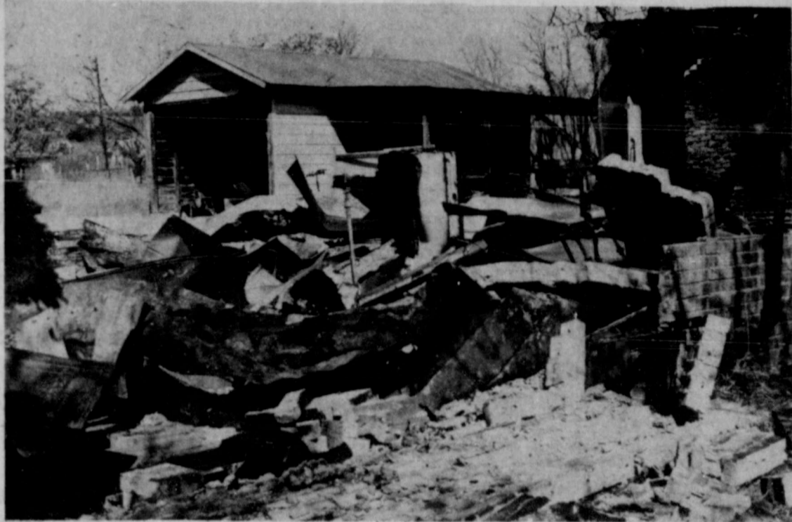
A TWISTED MASS of tin, brick and steel is all that remained of the Jerry Dellis home in Goldthwaite after a fire destroyed it last Thursday night.
