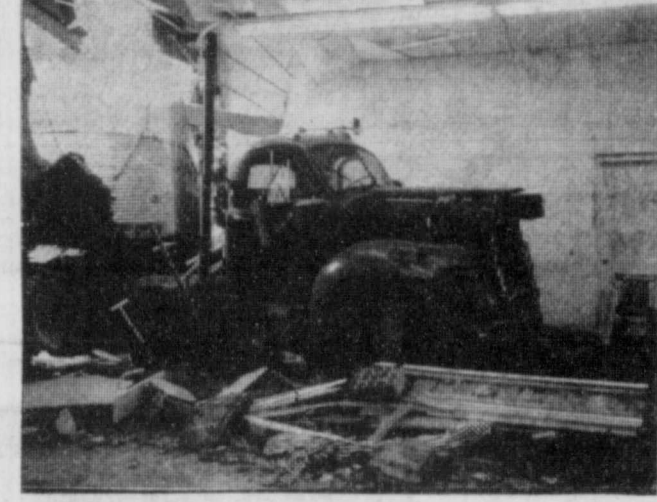
INSIDE VIEW —Here is shown the tractor, of the semi-trailer grain truck, after it came to a stop about 12 feet inside the Youth Center.
