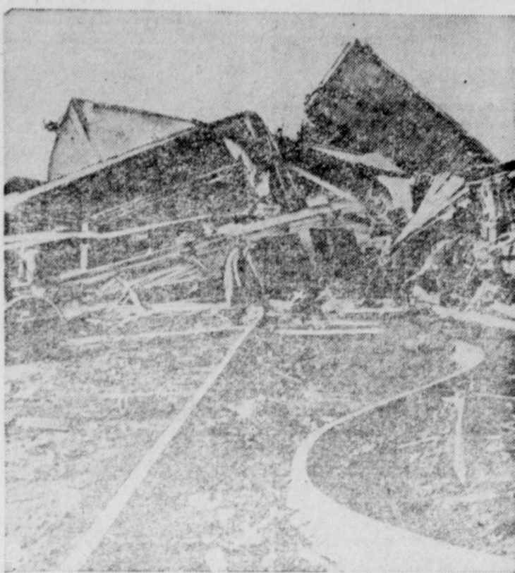
WORKMEN FACE a tough problem as they start clearing the tracks of wreckage, after 38 cars of an Omaha freight train piled up after being derailed near Menominee, Mich. Only the conductor was injured.
