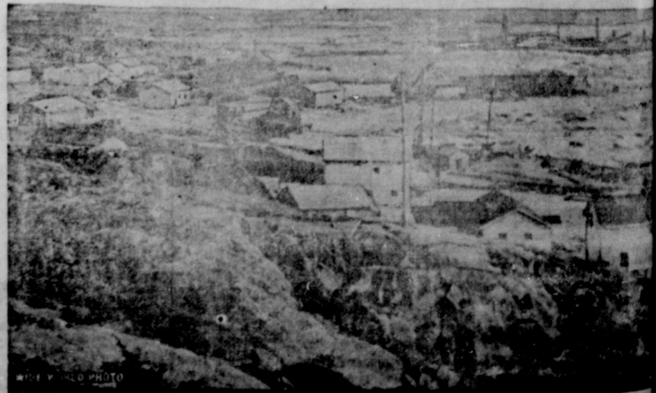
Construction camp at Churchill, on the west coast of Hudson bay, where Canada is building a port for the shipment of grain to Europe.
