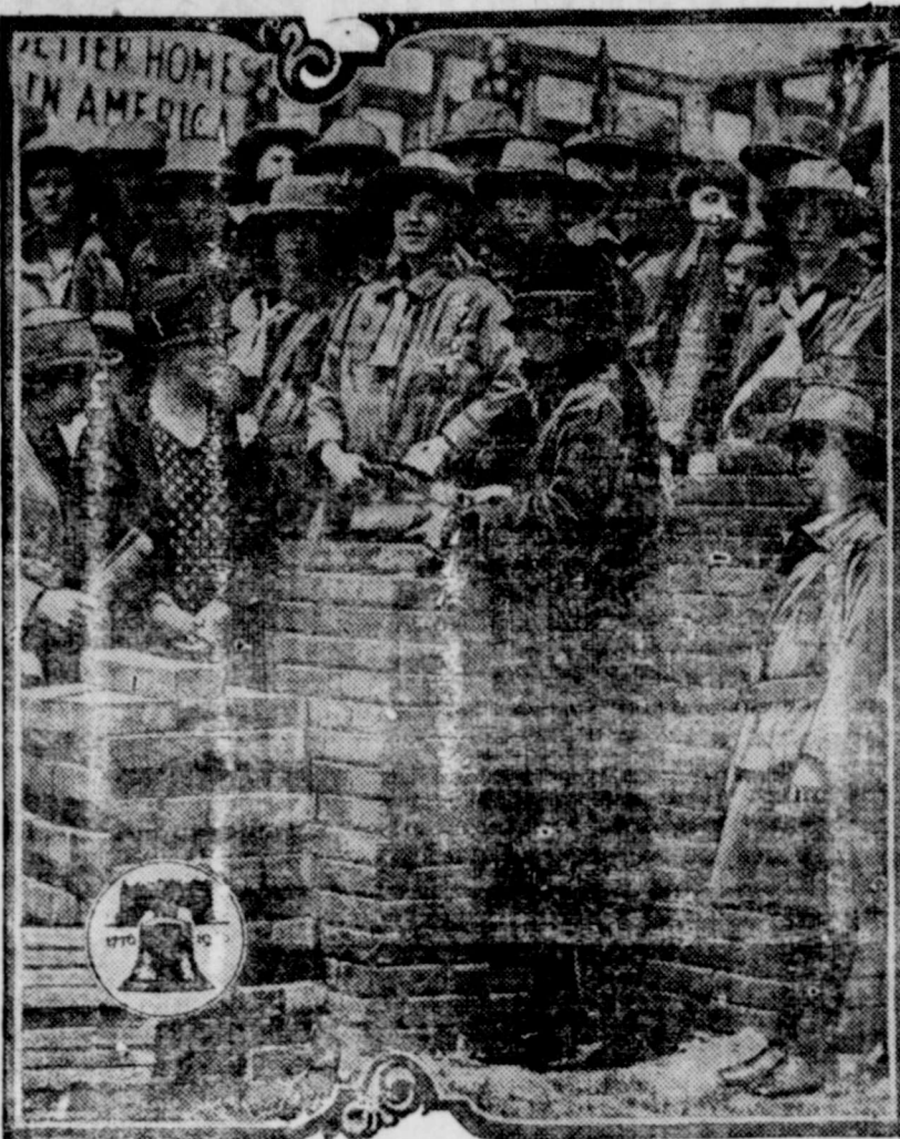
Mrs. Herbert Hoover, wife of the Secretary of Commerce in President Coolidge's cabinet, is shown laying the cornerstone for the model home being erected by Better Homes in America organization at the Sesqui-Centennial International Exposition, in Philadelphia June 1 to December 1 to celebrate 50 years of American Independence. Opposite Mrs. Hoover stands Mrs. Vance deCormick of Harrisburg. The Girl Scouts grouped around the women will operate the house.
