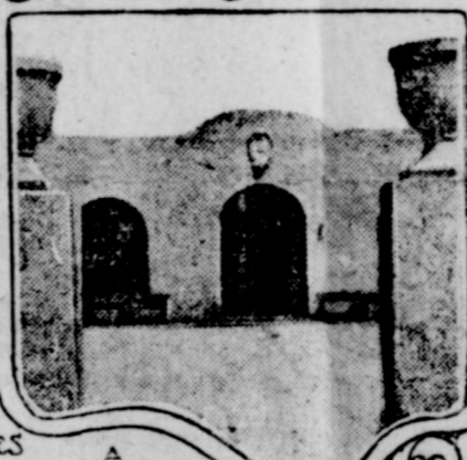
A RECREATION PATIO BETWEEN MENS AND WOMANS BLDG.
