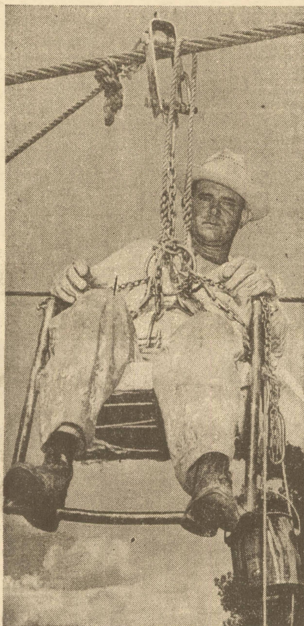
Invented by members of Lone Star Gas paint crew this boatswain's chair enables them to paint pipeline suspension bridge rods in less time than they used to require. It was designed primarily for the safety of the painter.
