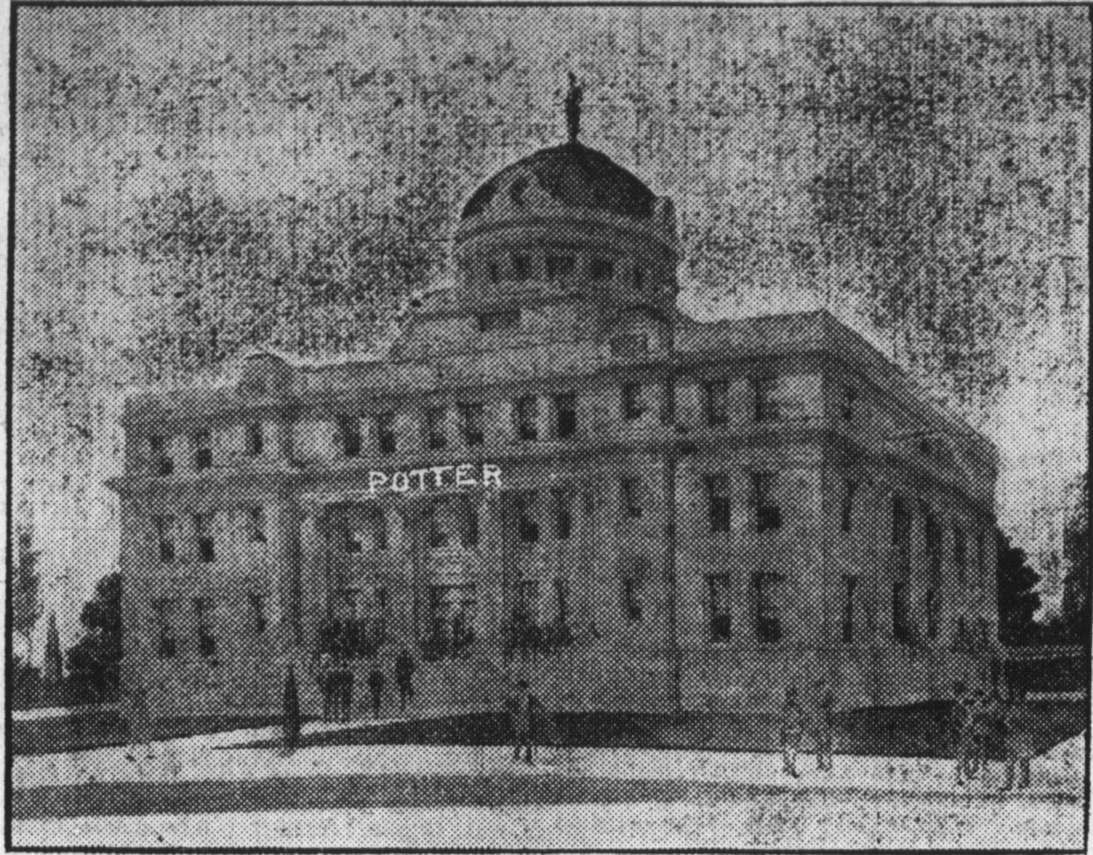
New Potter County Court House—J. J. Holt, Contractor, Amarillo.
