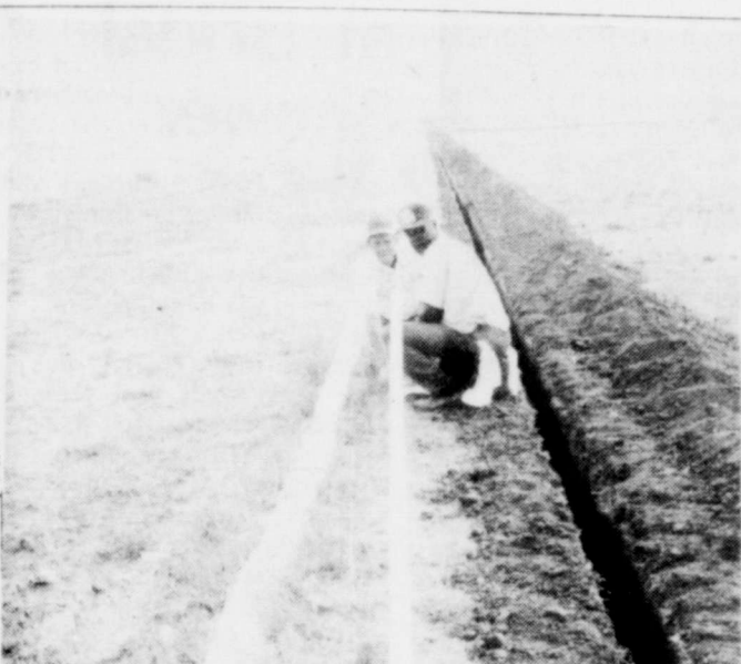
INSTALLING PIPE AT SCHOOL —Charlie H. McDaniel, left, who received the contract to install over 1400 feet of 2 inch pipe for watering the local school campus, is pictured above as he and Felix Walton, right, laid some of the pipe for the RC&D project for beautifying the local campus.
