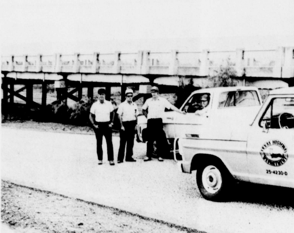
LAST TRIP OVER —Leroy Gibson, rural mail carrier for Hardeman and Foard Counties, makes the last official trip across the old bridge over the Pease River between the two counties. Here he chats with members of the Texas Highway Department staff who were to begin Tuesday demolishing the old bridge to make room for a new one to be constructed this winter. A detour bridge route over the river is shown here just to the east of the old bridge and will be utilized by traffic until the new bridge is completed sometime next year.
