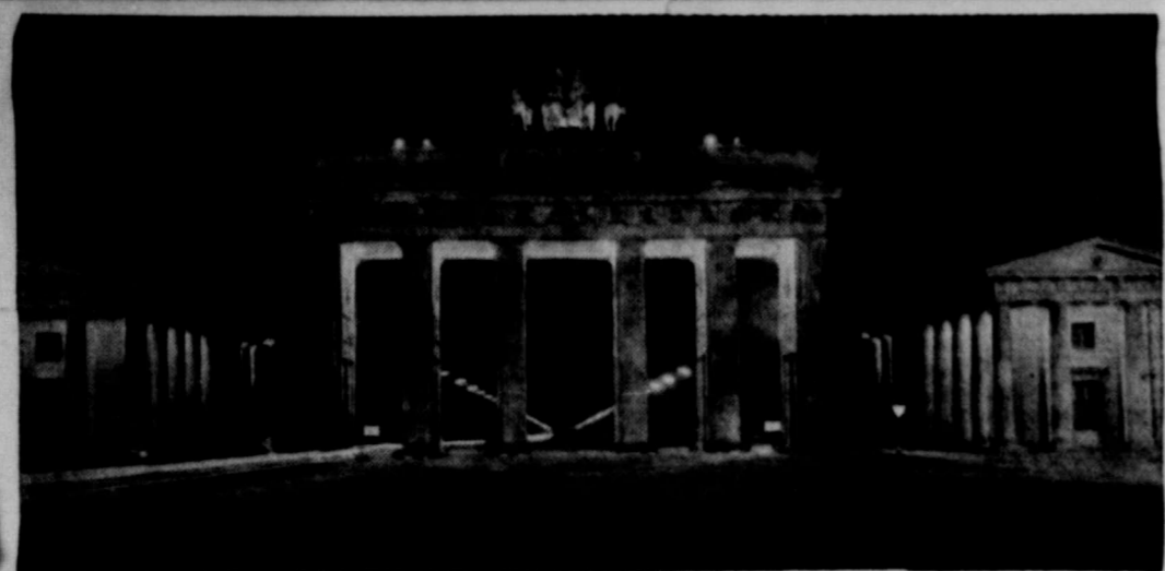
GATEWAY FROM DARKNESS —Floodlights add to the cold loneliness of this scene, a time exposure of the Brandenburg Gate in East Berlin, as seen from Red-dominated territory. The famed structure is located just across the border from West Berlin, and lights in background stretch into the Western-controlled portion of the beleaguered city.
