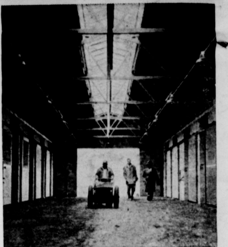
DE LUXE HORSE HOTEL - Carpeted with 10 inches of packed dirt over four inches of gravel, portion of horse barn pictured above, is only a small part of a de luxe horse hotel for the elite of the equine world now under construction at Yonkers Raceway, Yonkers, N.Y. Eight 84-stall, two-story barns will be in the group. "Apartments" on second floors will be staggered so that guests walking about above won't disturb the temperamental occupants of first-floor "suites." Ramps will lead to the second-story accommodations. Cost of the project: About $2,700,000.
