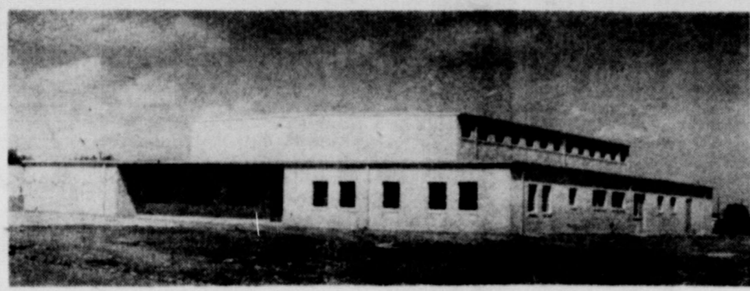
The new $70,000 armory, home of company I, 142nd infantry, was formally dedicated Saturday and many Ballinger citizens were present. In addition to being an armory, the building will also be a community center and already several gatherings have been held there.
