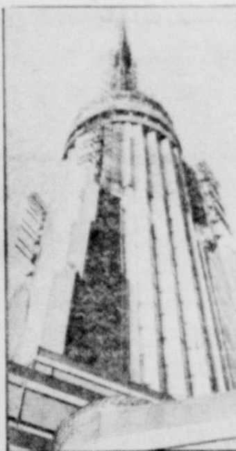
HIGH "SEE" —Television antennae atop the Empire State Building in New York City mark the highest point to which man has ever raised a structure—1472 feet above ground level. More than 15 million persons live in the four-state area reached by the multiple-station broadcasting equipment.
