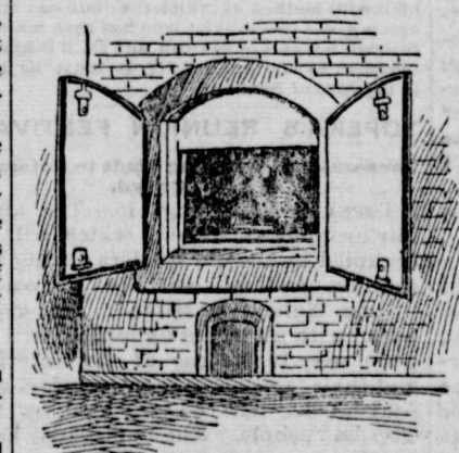
FURNACE IN CHICAGO CREMATORY.
