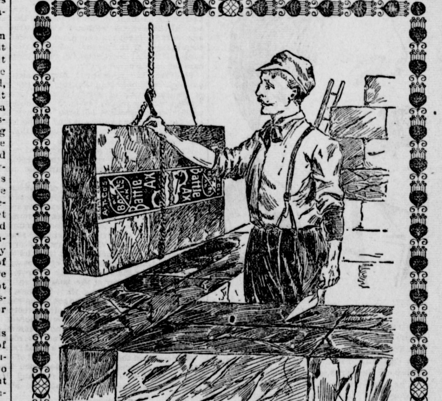
"A Good Foundation."
