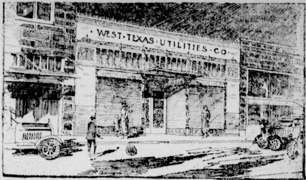
New Office Building Being Erected by the West Texas Utilities Company in Ballinger.
