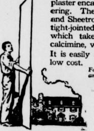
Sheetrock is genuine gypsum wall plaster encased in a protective covering. The patented joining edge and Sheetrock Finisher insure flat. tight-jointed and smooth surfaces which take wall paper, paint or calcimine, with or without panels. It is easily and quickly put up at
