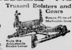
On the front bolsters of Thornhill wagons are heavy iron plates running along top and bottom-connected by rivets that run clear through the bolster. Strength and lightness are combined. Rear gears are strongly ironed. There are braces on both top and bottom that extend the full length of the
