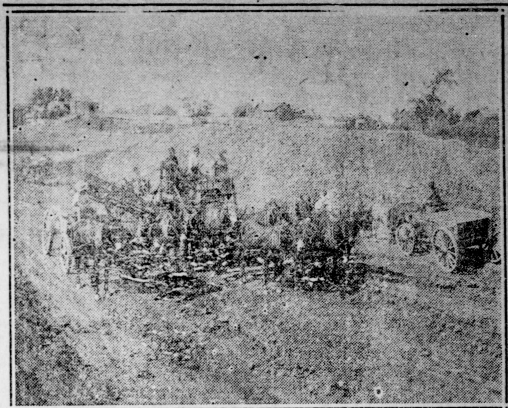
Giddings, Texas: The Houston and Texas Central Railroad is constructing a line between here and Stone City. The route crosses the Santa Fe tracks near Caldwell and the grade is being lowered thirty feet to make the subway. The above scene is a view of a construction gang at work at this point on the line. There are nine railroad projects under construction in this State at present. When completed these lines, together with seven proposed routes will give Texas an additional 1,577 miles of trackage. Four interurban lines are being built and five routes are under contemplation.
