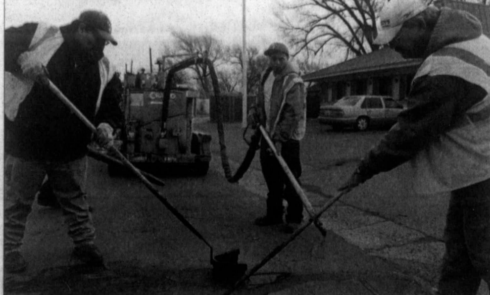
staff photo by David Bowser Ben Ponce (center) fills cracks in the pavement with hot tar while Peter Solorzario (left) and Zach Stillwell smooths it out in an effort to repair Pampa streets before the next winter front blows down from the north.
