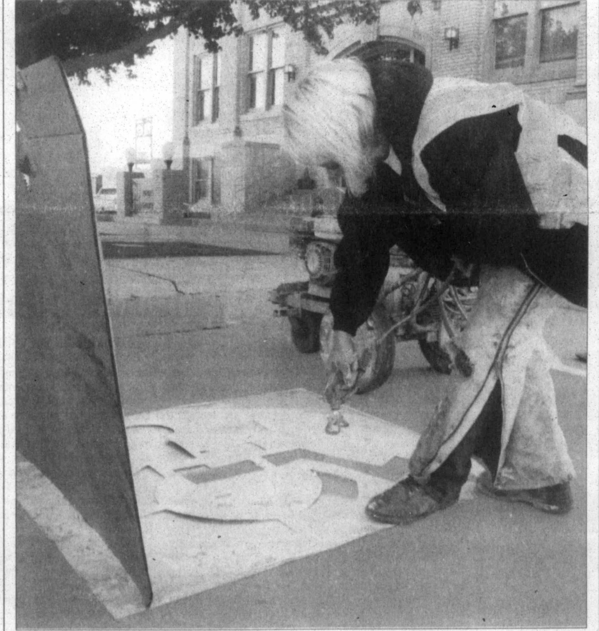
Ruth Williams of the city's street department spray stencils a handicapped parking space at Pampa City Hall today. staff photo by David Bowser
