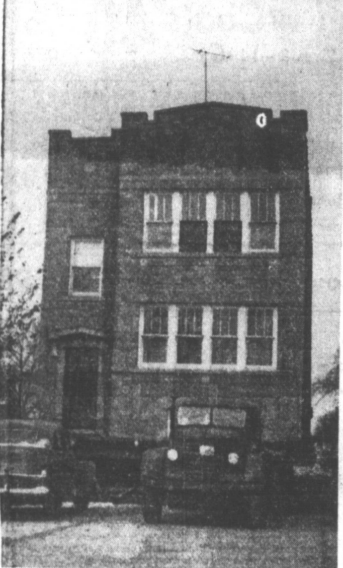
MUSIC ON THE WAY —Housekeeping went on as usual when the Henry Traum family had their two-story brick apartment building rolled down a street to a new location in Chicago. A temporary oil stove was rigged up and an electric line tied into a neighbor's line box kept appliances going, including the TV set. A new superhighway cloverleaf forced this move.
