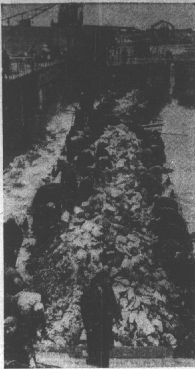
FINGERS IN THE DIKE —A Dutch "dike army" is shown in action on Schouwen Island, closing the last gap in their only defense against the seas that have so often swept over their land. Huge caissons have been sunk, security walls erected and rocks were carried by hand to complete the barrier. Even last winter's floods caused widespread damage and misery.
