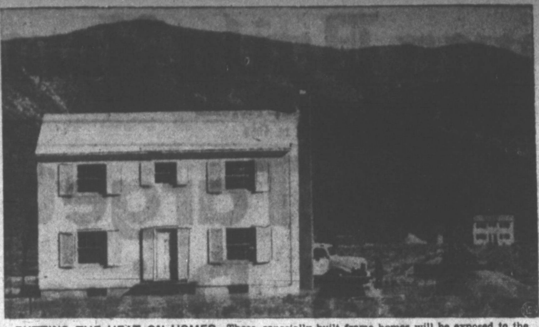
PUTTING THE HEAT ON HOMES—These especially built frame homes will be exposed to the heat and the blast of an atom bomb detonation at the Las Vegas, Nev., Atom Proving Grounds. The homes, completely furnished, contain mannequins as the "victims" and will play an important part in the Federal Civil Defense phase of the test.
